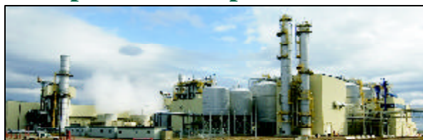
Husky Energy's 130-million-litre Saskatchewan wheat-ethanol plant
